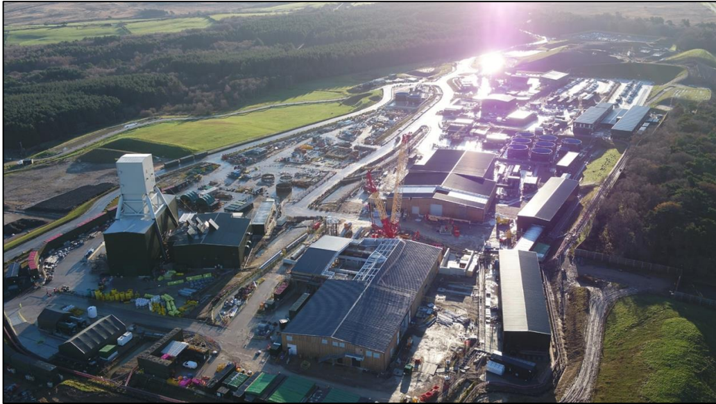
Figure 1.3 Woodsmith Project: Minehead Site, March 2022
