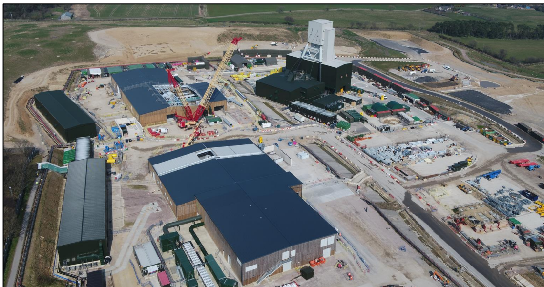
Figure 1.4 Woodsmith Project: Minehead Site, March 2022
