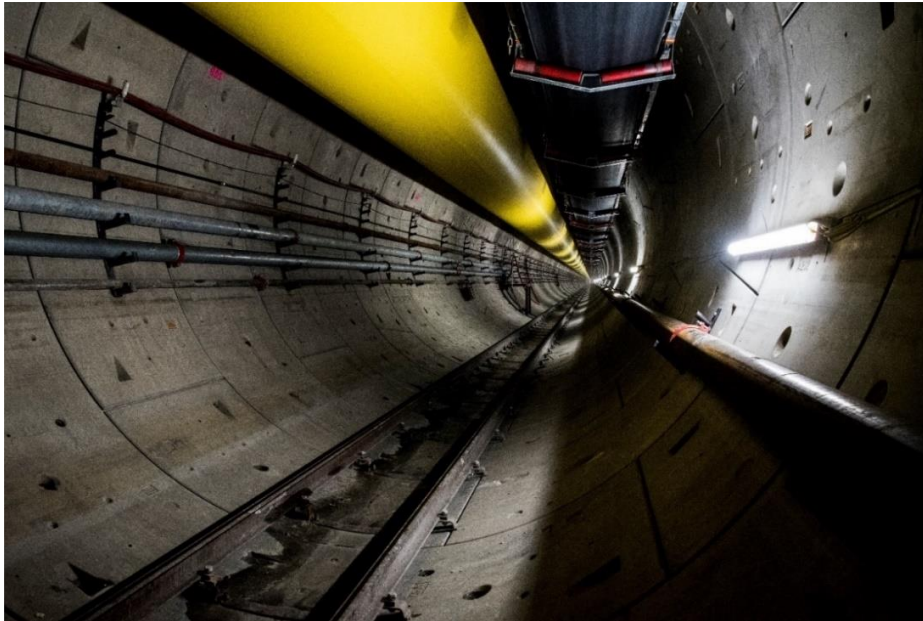
Figure 1.7 Woodsmith Project: MTS Tunnel
